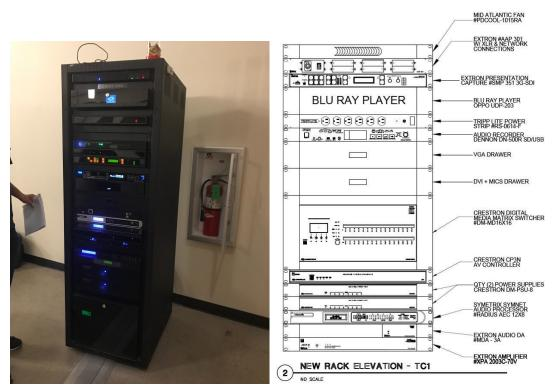
Figure 4: AV rack in Giedt Hall (left) and device breakdown for a typical AV rack from building drawings (right)
