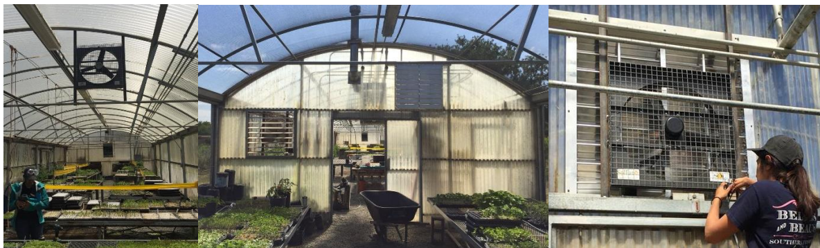
Picture 1: Middle-fan installed.
